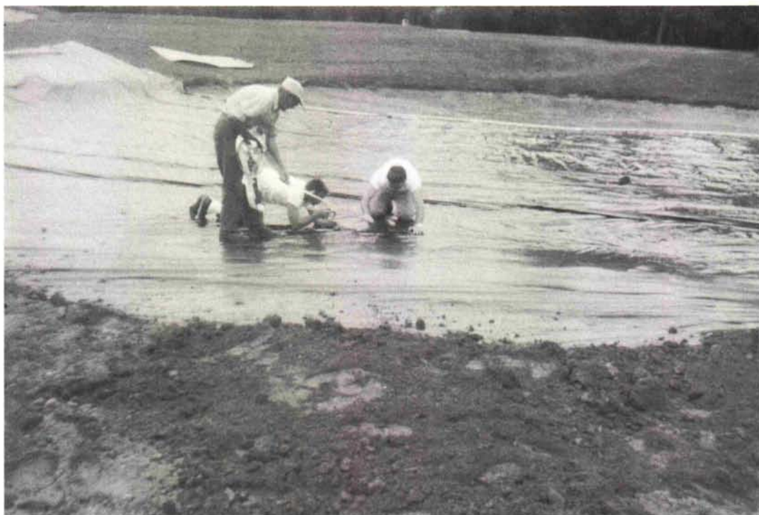
Laying plastic sheets. Partial covering with soil in foreground.
