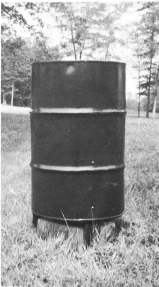
Another way of protecting automatic controllers is to use a large steel barrel over the unit to keep out harsh weather (Figure 4).
