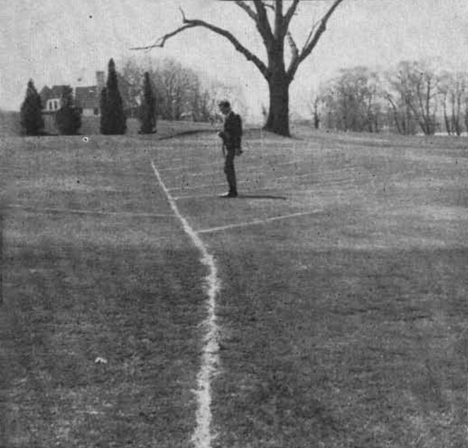
Bill Madigan of Forest Lake Country Club in Detroit (left) stands amid "herringbone" slit trench design on one of his greens. Al Bunn, Illini Country Club, Springfield, Ill., (right) shows slit gravel trenches draining into a creek from low fairway area
