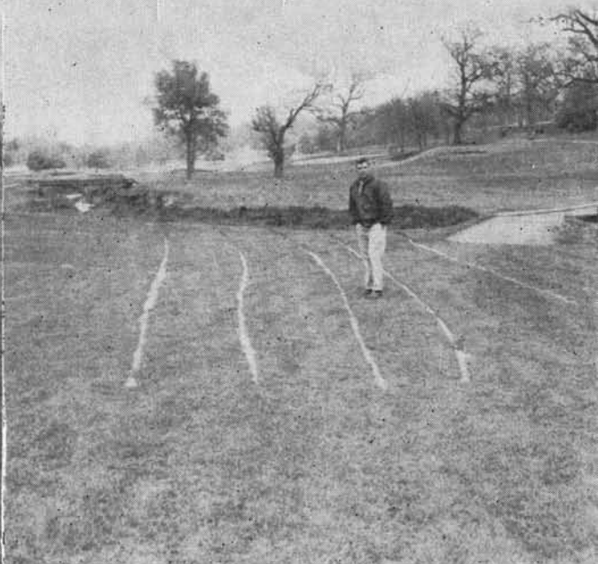
Bill Madigan of Forest Lake Country Club in Detroit (left) stands amid "herringbone" slit trench design on one of his greens. Al Bunn, Illini Country Club, Springfield, Ill., (right) shows slit gravel trenches draining into a creek from low fairway area
