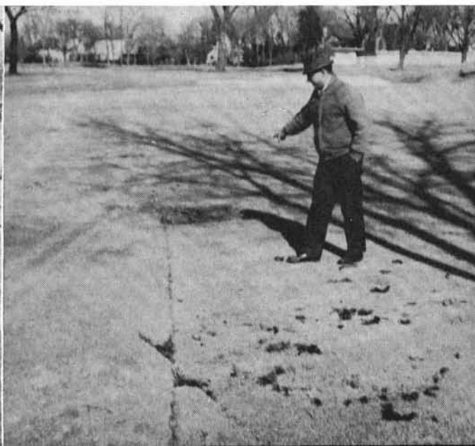
Use of chain saw (left) is convenient way to make tiny slit trenches in green. Fairway slit trenches (right) are wider and deeper.
