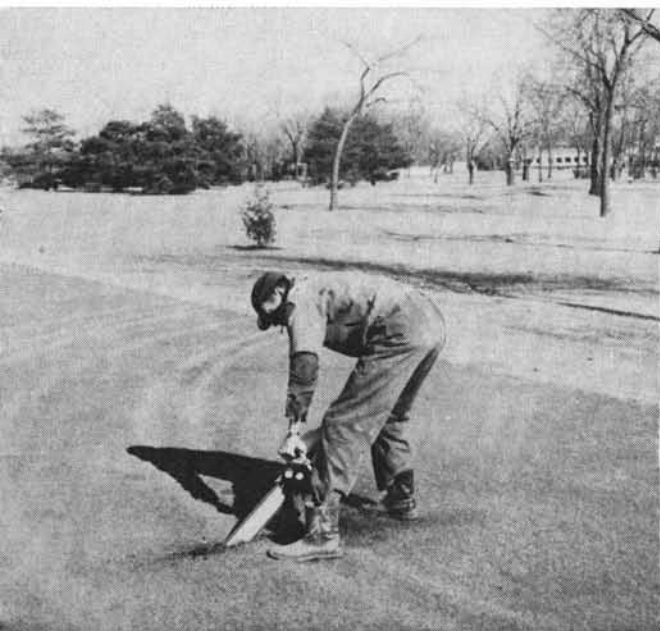
Use of chain saw (left) is convenient way to make tiny slit trenches in green. Fairway slit trenches (right) are wider and deeper.
