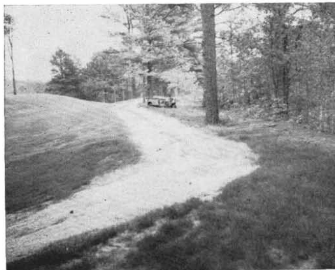
The drain ditch is covered and the metal pipe in underground. Major floods can go to the extreme left if pipe is too small.
