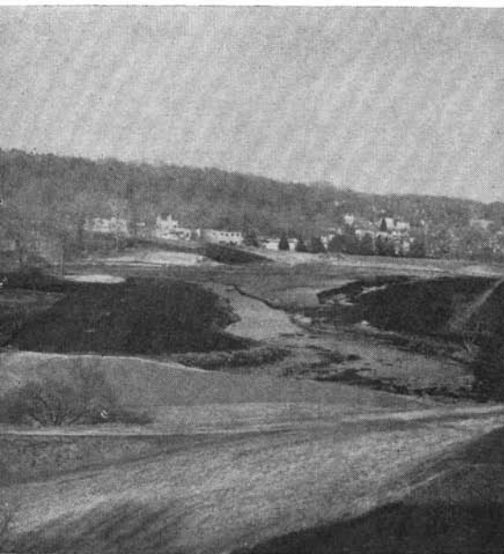
Figure 1 - Not a river bed, just a water development project at Scarsdale Country Club, Hartsdale, N. Y. Improvement included realignment of several holes which was made possible after dredging for improved water supply for irrigation. A large shallow pond covered the area previously.
