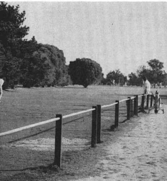
Fixed fences are a help in traffic control, but note worn area on the tee at the narrow fence opening. Entrance was purposely narrowed to keep hand carts off the tee.
