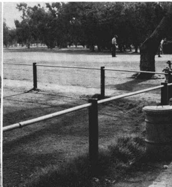
Fixed fences also present a mowing problem. If the fence posts were set in a 'sleeve' and were moveable, mowing and entrance problems would be overcome.
