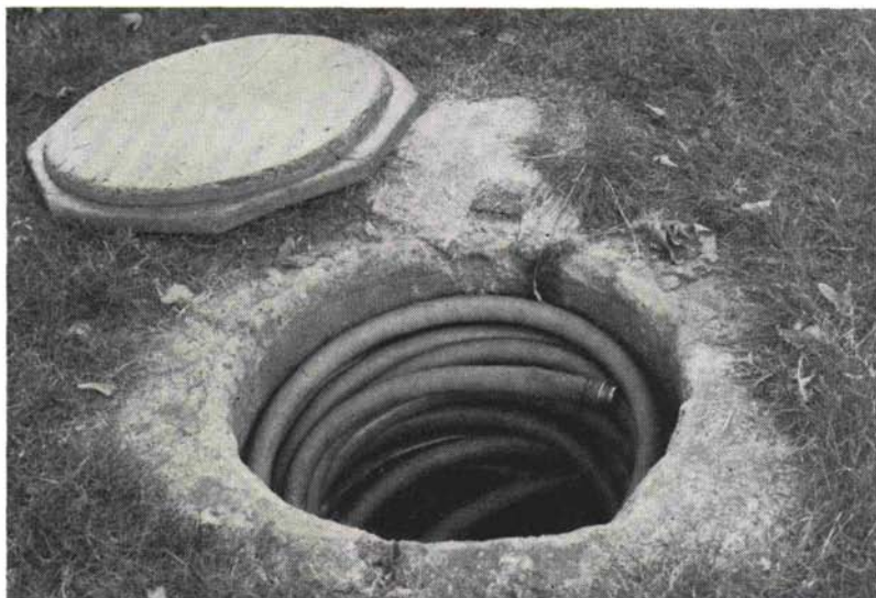
Supt. Bob Peters of Gulph Mills Golf Club, King of Prussia, Pa., constructed boxes of cement to store irrigation hose in close proximity to each green. Some are constructed so they can be padlocked.
