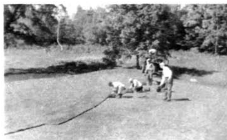
2. Laying the sod—note light raking by Mr. Baskin before sod is laid.
