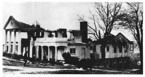
The fire that practically destroyed this three-story wooden building had been burning more than an hour before discovery by a passing motorist. Originating in the basement, it had spread throughout the first story by the time firemen arrived. The building was protected by a rate-of-rise type automatic fire alarm system but due to the fact that it was not connected to the Fire Department and had no outside alarm, its performance at this crucial time was of no value.
