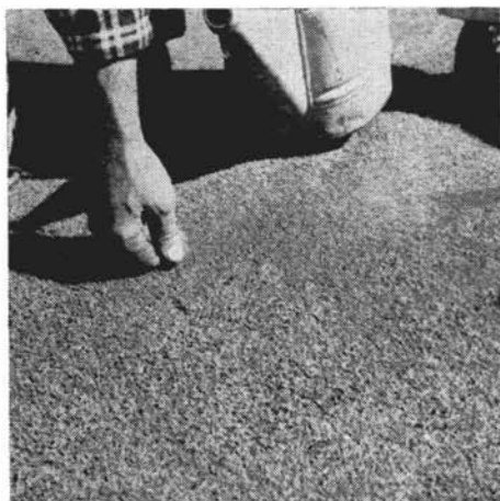
Perimeter is firmed as plug is watered.
