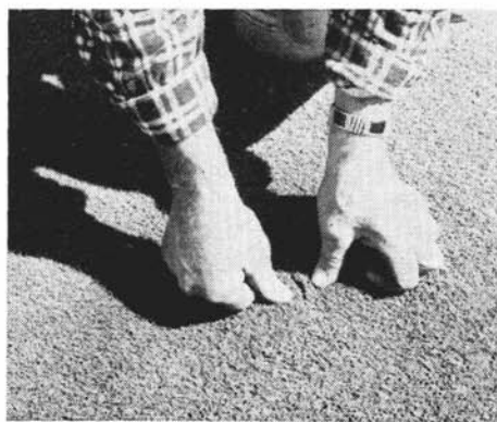
Edges are separated to release grass blades forced into the slit around perimeter.
