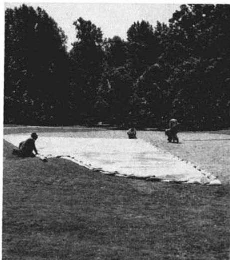
Fig. 4. Sand-bagging the edges of the plastic cover.
