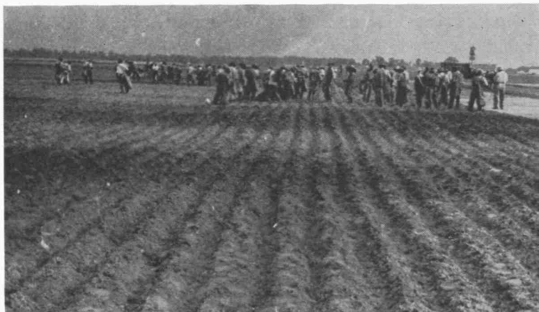
Sprigging Bermuda grass on a southern airfield. Note the "army" of men necessary for large scale planting by the hand method. Bermuda grass sprigs are being placed in furrows by hand, after which they will be covered. Some mechanical planting method would not only greatly reduce the time required for this operation, but would prevent the drying out of sprigs before covering.
