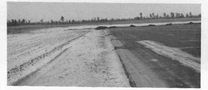
Trench 10 feet wide at the edge of an airfield runway excavated in preparation for "mucking." A 4 to 6-inch layer of muck is used to fill the trench. Natural vegetation growing in the muck is expected to produce a dense cover along the edge of the runway. The muck has already been placed in the trench in the background.
