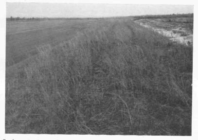
Ten-foot strip of muck which has been in place along edge of airfield runway approximately one year. Note the dense growth of natural vegetation on this strip which prevents soil from washing onto the runway. Often the vegetation obtained in this way will not survive the dry conditions on airfields since it is usually brought in from low swampy areas.
