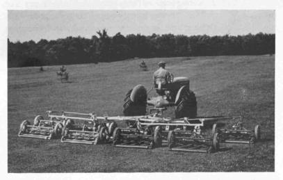
Reel type gang mowers may be effectively used on large open turfed areas. This type of mower is operated at a higher speed and is much more effective in controlling weeds than the ordinary sickle-bar type. The time required for mowing may be kept at a minimum by using 7 or 9 unit gangs of these mowers.
