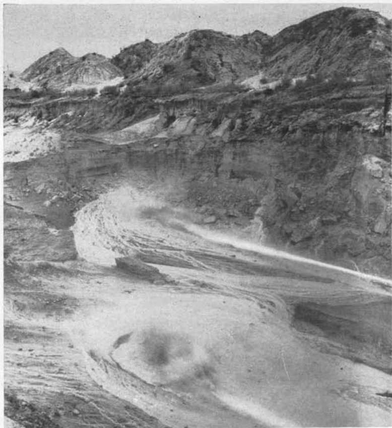
Mining of phosphate rock by means of the hydraulic method in Polk County, Florida. Note jets of water coming in from the right.
