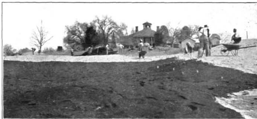
Use of sand and peat in improving the structure of a clay soil on the course of the Augusta National Golf Club. The area to be improved was first covered with a layer of sand (above) and this in turn was covered with a layer of peat (below). These layers were then thoroughly worked into the surface soil.
