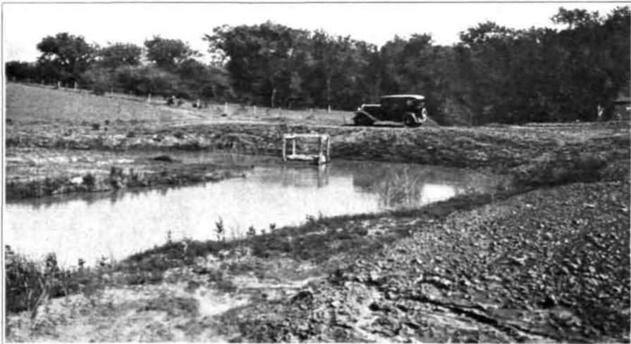
Large soil-saving dam in use on the Federal and State Soil Erosion Experiment Station near Bethany, Mo. A fill of more than 4 feet of soil has already formed above this dam
