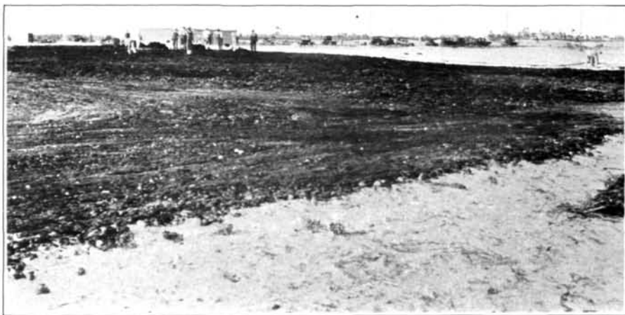
Covering sand with layers of marl and muck in constructing fairways at Boca Raton, Fla. The materials were later mixed by discing. This process is an expensive one but on some courses it has been considered advisable in order to make the soil more firm and better able to retain water and plant foods.
