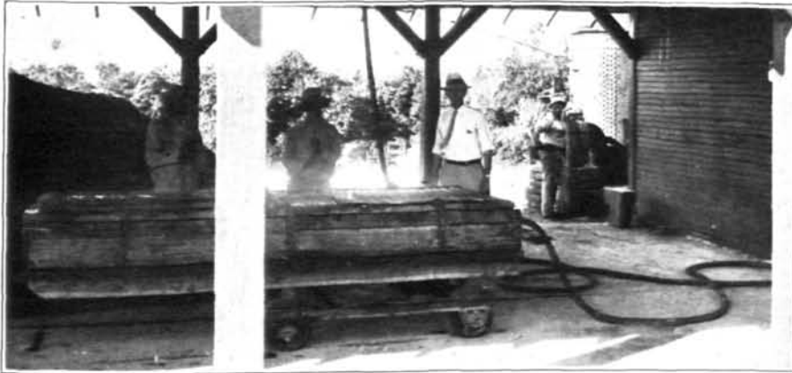
Soil and compost sterilizer constructed and used by the Gulf Stream Golf Club, Delray Beach, Fla. By the use of this apparatus the material is steamed, at a small cost, so as effectively to eliminate injury to putting greens by nut grass, pennywort, and various other turf weeds.
