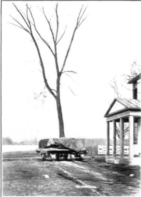
A 24-inch elm tree being moved one-third of a mile on house rollers
