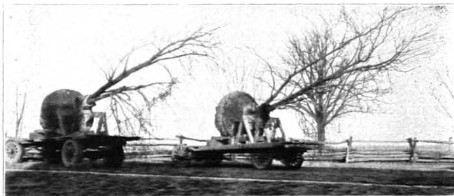
In moving large trees for transplanting a trailer made from an old truck chassis is an excellent carriage.
