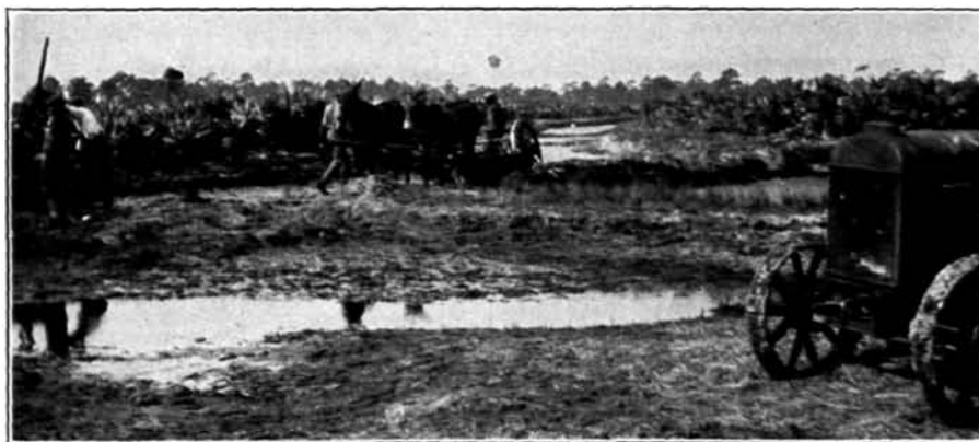
Digging a wide, open ditch with a wheel scraper on the side of a low fairway in Florida. The fill is being used to raise the fairway and to build the green and tee.
