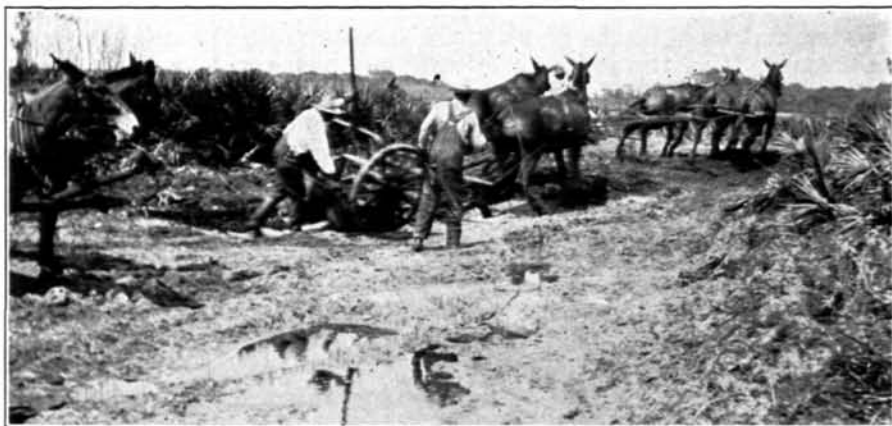
Snatch team loading a wheel scraper.
