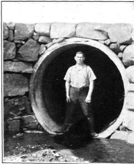
The 76-inch pipe under the fifth and tenth fairways.
