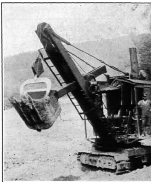
Steam shovel grading hill on the first hole
