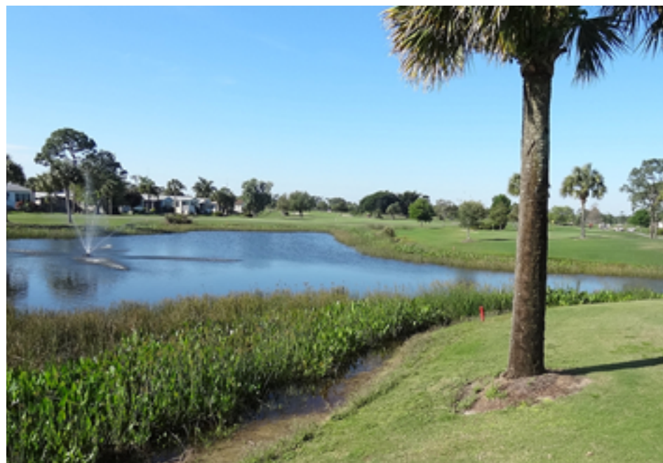
A golf course pond built with a littoral shelf extending out from the pond's edge provides an area for emergent plants that create a buffer, provide habitat for aquatic organisms, and help reduce bank erosion.
