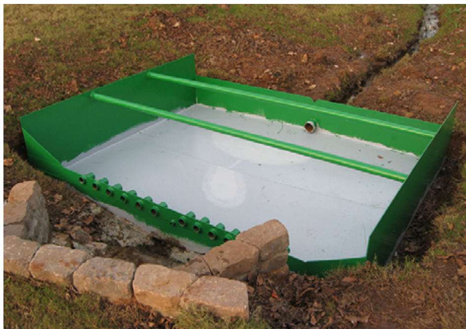
Figure 1. The uncompleted phosphorus removal structure shown during construction.
