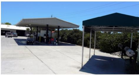
Covered equipment wash/fuel areas improve staff morale, reduce fuel evaporation, and lengthen the useful life of tanks and hoses. These areas are staged so that equipment may first be blown off with compressed air (foreground) before washing/fueling. Equipment can then be inspected by equipment managers (background) or stored.
