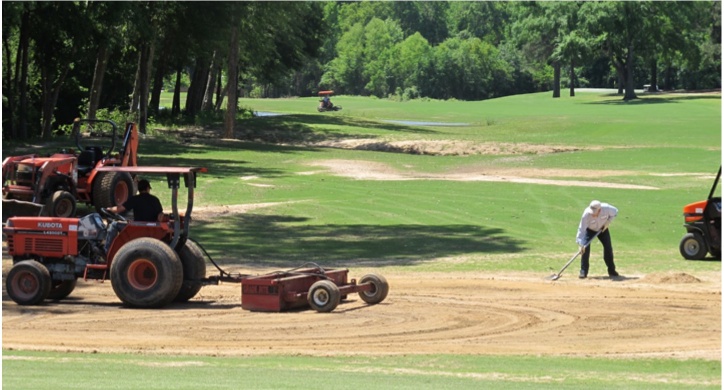
Heavy equipment may be required to unearth buried turf from the soil deposited by a flood.
