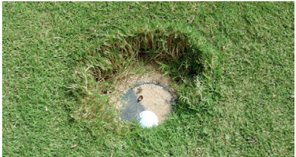
Time spent raising low irrigation heads will improve coverage uniformity and help maximize life expectancy of the irrigation system.
