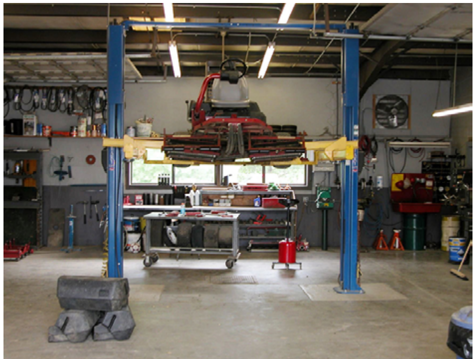
A properly equipped maintenance complex accommodates safe and efficient servicing of equipment, which improves performance and life expectancy.
