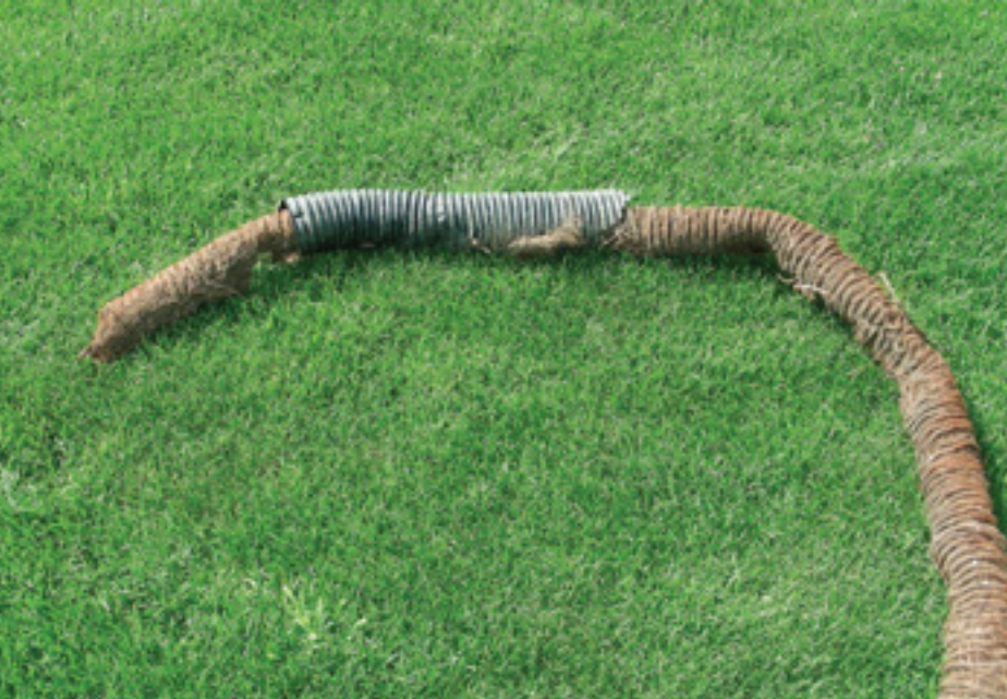
At times, tree roots can completely engulf and damage a drain line.
