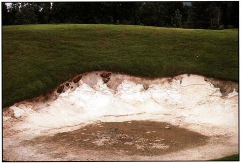
Flashed sand faces are dramatic architecturally, but when surface water is allowed to run into a bunker with a flashed sand face, washouts are inevitable.
