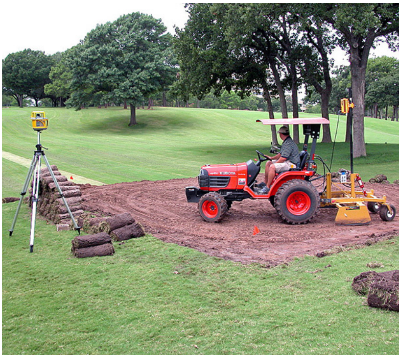
Laser leveling of tees is easily accomplished in-house if proper equipment is obtained.
