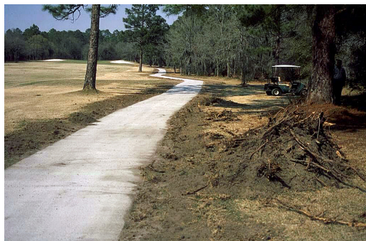
Cart path additions must be installed to the proper grade. Addressing tree roots should be a major concern for long-term success.
