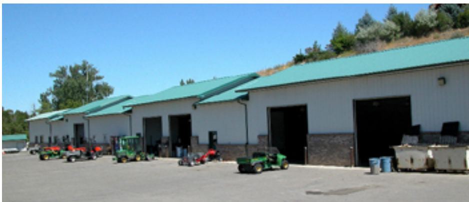
Modern, well-designed maintenance facilities provide sufficient area for equipment servicing and storage as well as administrative duties and safe working conditions for employees.
