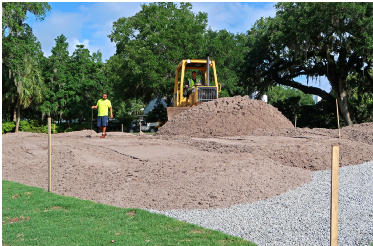
Selecting and installing the rootzone mixture according to the USGA Recommendations is critical for effective moisture management. The physical properties of the rootzone mix ensure adequate water retention and sufficient drainage.
