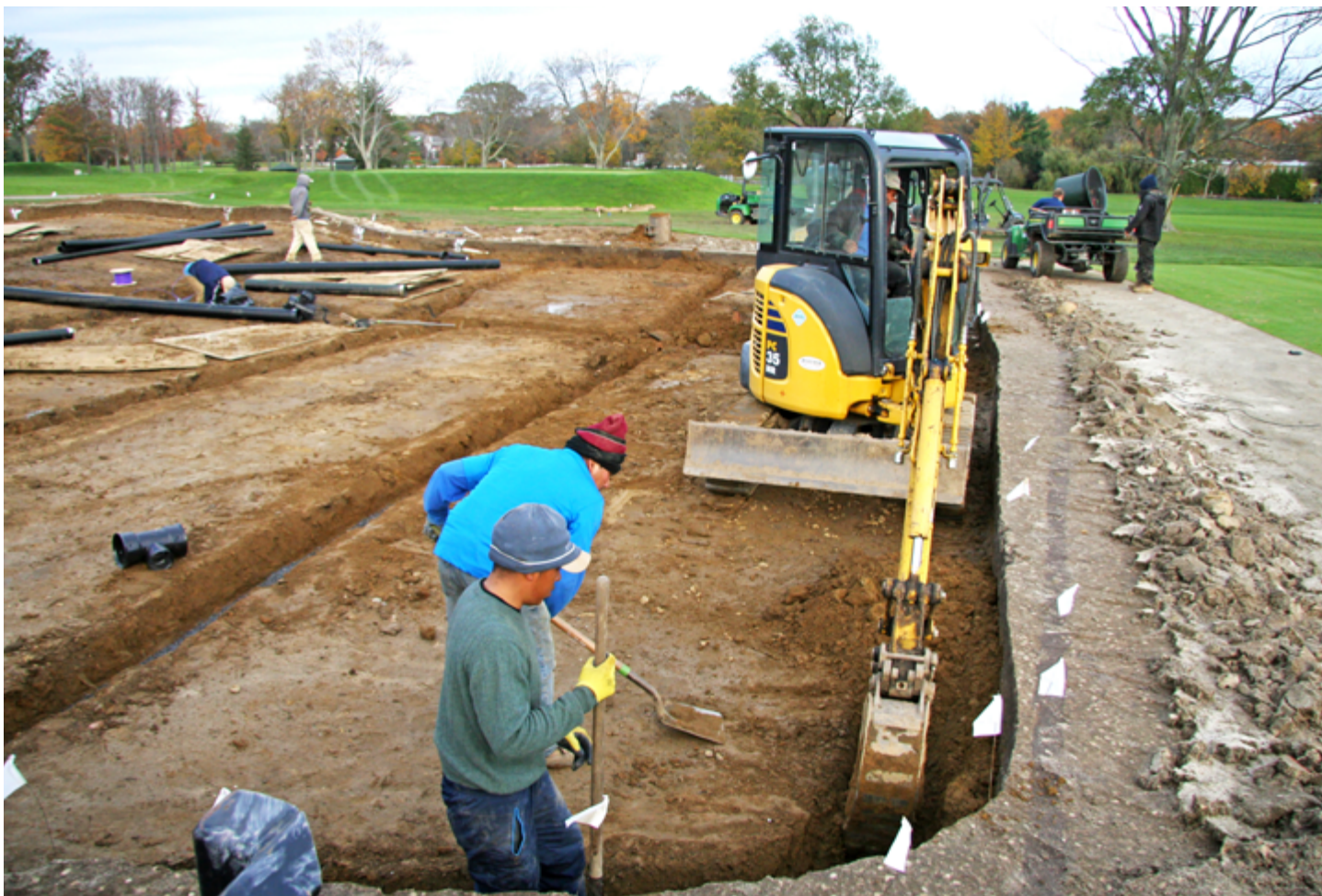
The drainage principles of the USGA putting green are one of the features that sets it apart from other construction methods.
