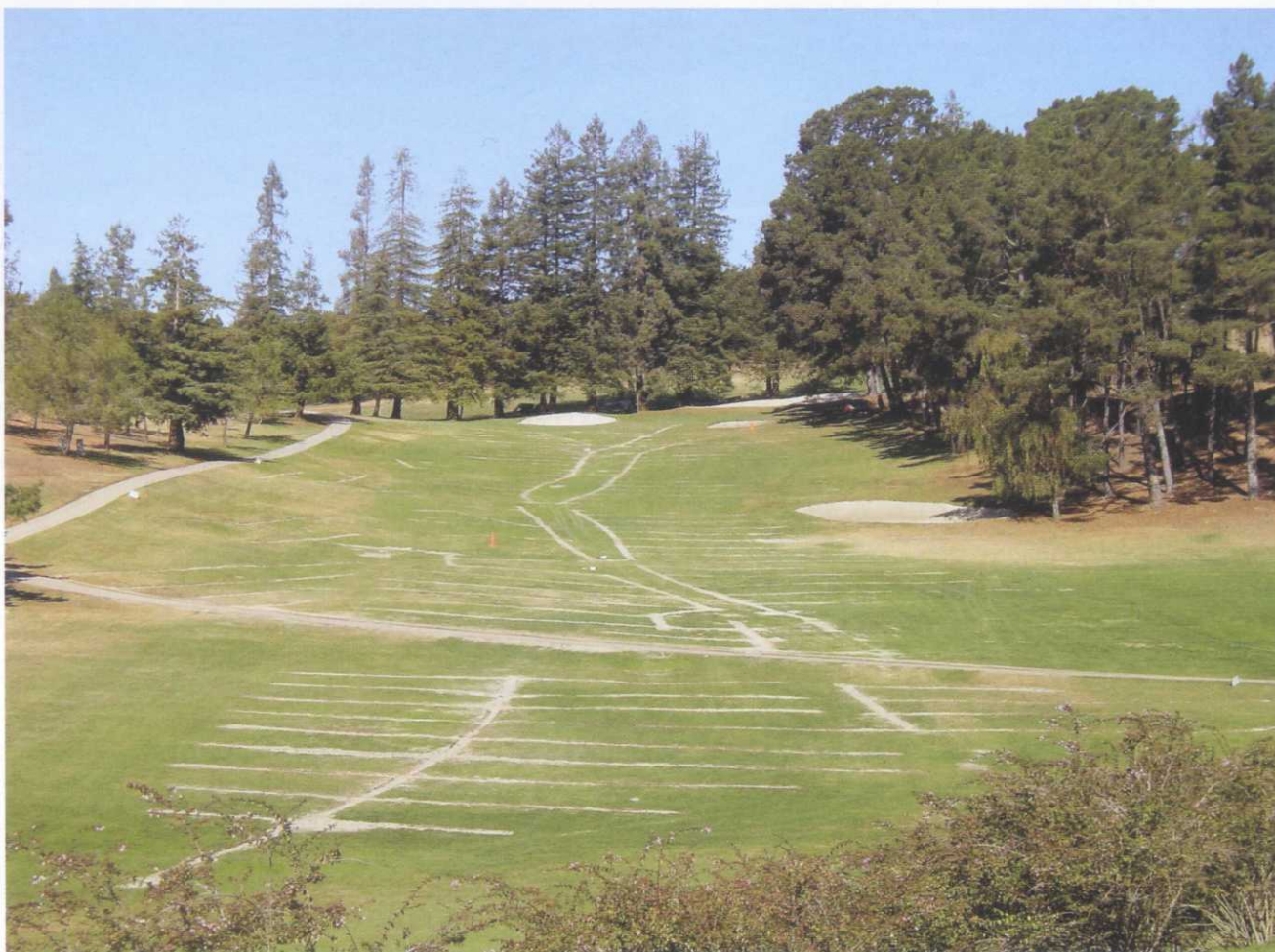
Seepage drainage design is critical for success of a drainage project. Seepage line installation runs parallel to the flow of the incoming drainage water, either parallel or perpendicular to the irrigation system, and is set up to facilitate the fastest movement of the spoils.
